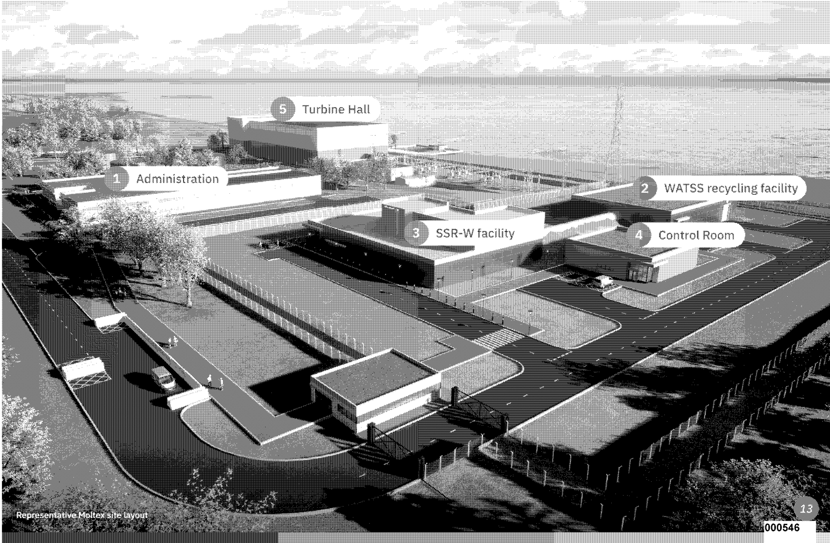
Point Lepreau: A national project in New Brunswick
