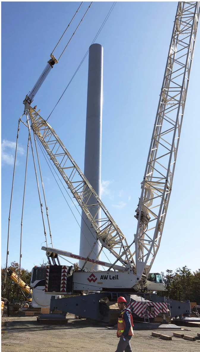
Wisokolamson Project construction, near the Village of Riverside-Albert, New Brunswick (SWEB)
