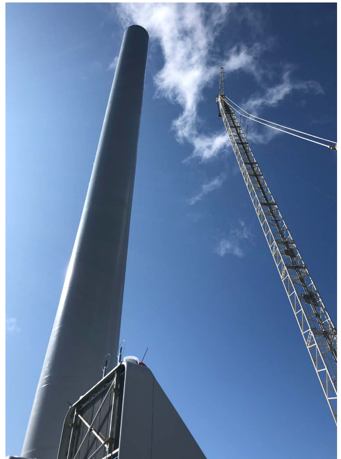
Wisokolamson Project tower construction, New Brunswick (SWEB)
