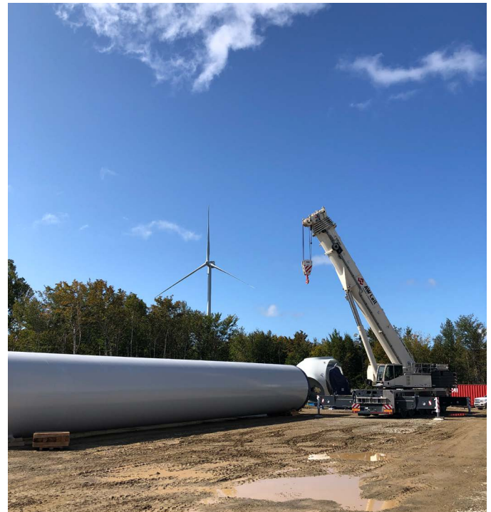
Wisokolamson turbine installation near the Village of Riverside-Albert, New Brunswick (SWEB)
