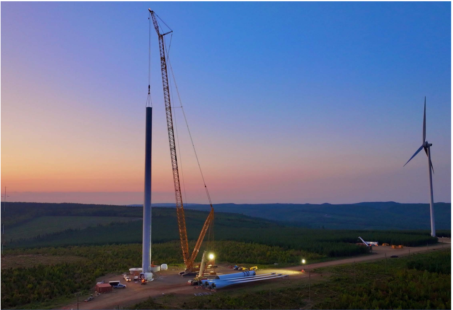
Neweg Project turbine tower construction, Kings County, New Brunswick (Natural Forces)
