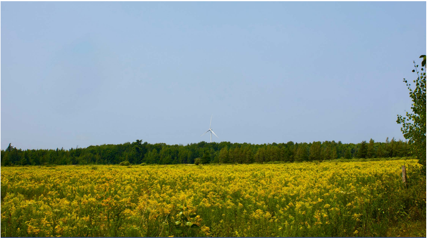
The sole turbine making up Pabineau First Nation's Oinpegitjoig Project in Richibucto, New Brunswick (Emma Fackenthall)
