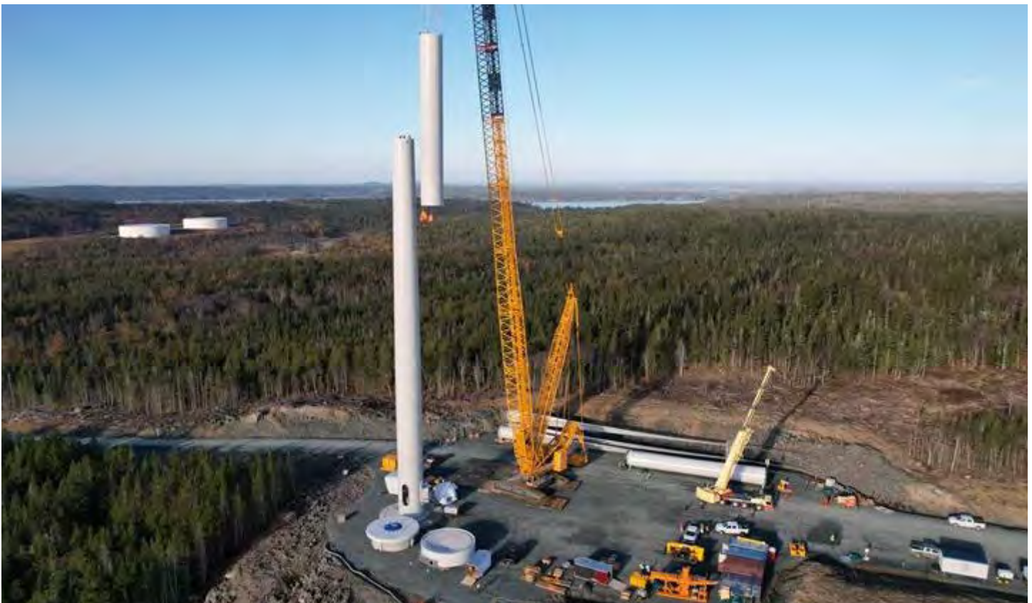
Construction of a Burchill Project tower, New Brunswick (Natural Forces)
