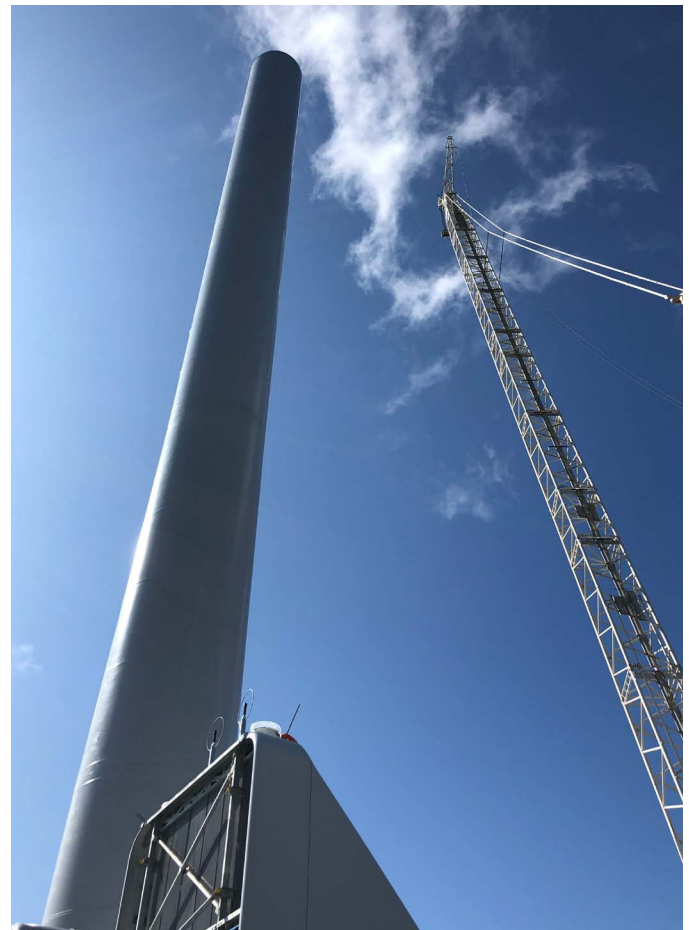
Wisokolamson Project tower construction, New Brunswick (SWEB)
